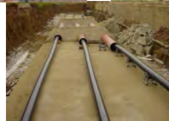
Buried cable system incl. junction structures
