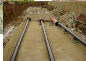
Buried cable system incl. junction structures
